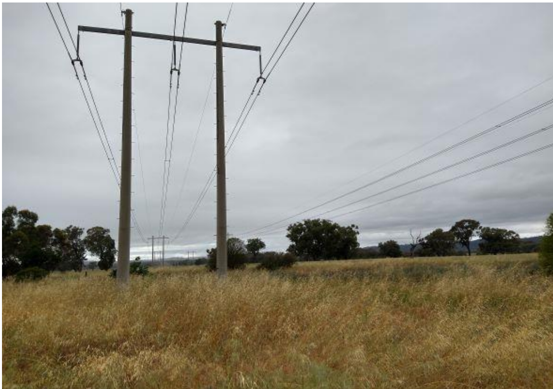
Photo 5 - Concrete pole supported power lines
